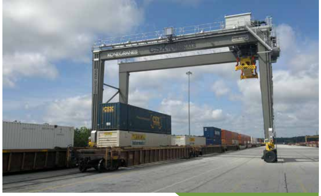
The CSX intermodal terminal at Valleyfield, Quebec, is but one example of the competitive tools the U.S. railways can mount to gain traffic at the expense of the Canadian lines, diverting it to their own and often superior routes close to the border.
