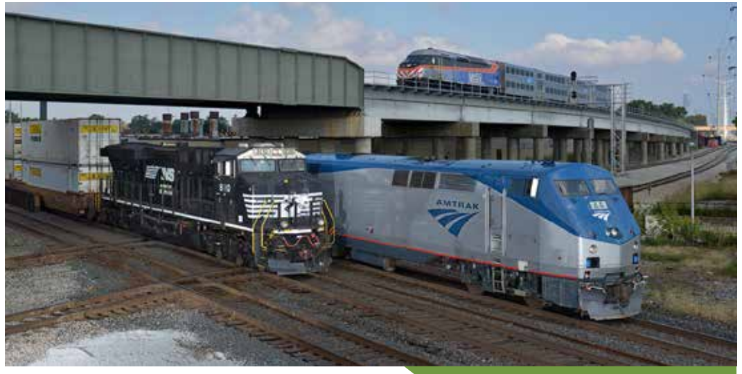
Chicago's Inglewood Flyover was constructed under a public-private partnership to bring benefits to Amtrak intercity passenger, Metra commuter and Norfolk Southern freight services. Photo courtesy CREATE
