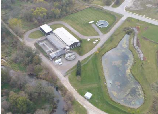
Figure 1 Thamesford WWTP Aerial Photo
