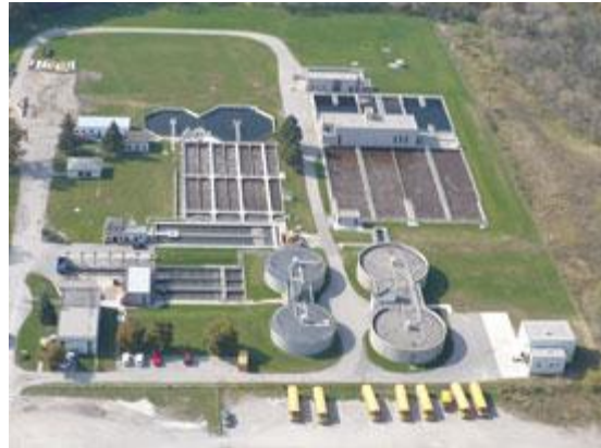
Figure 2 – Woodstock WWTP Aerial Photo
