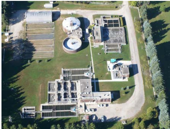
Figure 1 Aerial view of Ingersoll WWTP
