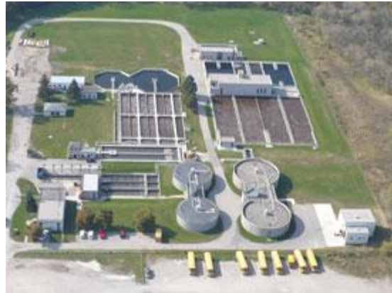
Figure 2 – Woodstock WWTP Aerial Photo
