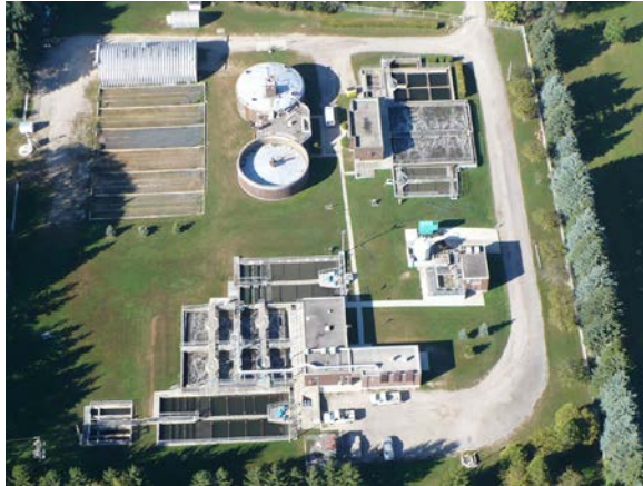
Figure 1 Aerial view of Ingersoll WWTP
