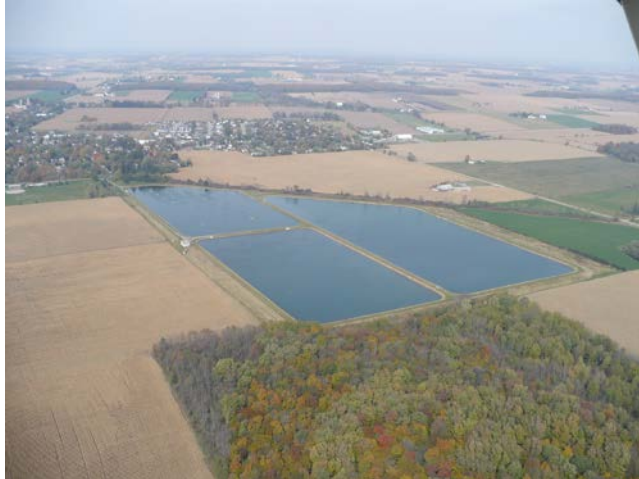
Figure 1 Aerial view of Tavistock WWTP (prior to recent expansion/upgrades)
