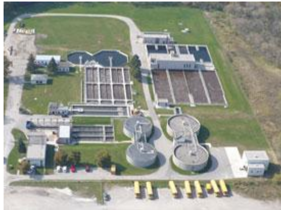
Figure 2 – Woodstock WWTP Aerial Photo
