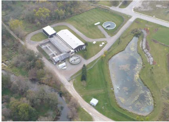
Figure 1 Thamesford WWTP Aerial Photo
