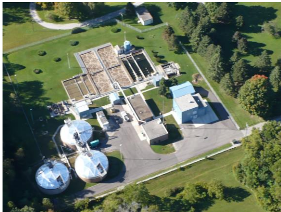
Figure 1 Tillsonburg WWTP Aerial Photo
