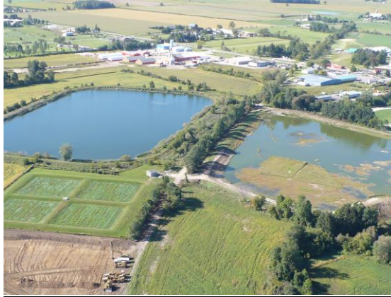
Figure 1 Aerial view of Norwich WWTP
