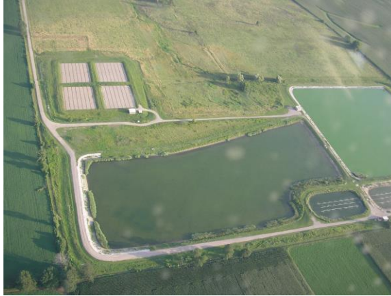
Figure 1 Plattsville WWTP Aerial Photo
