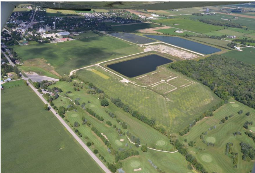
Figure 1 Aerial view of Tavistock WWTP
