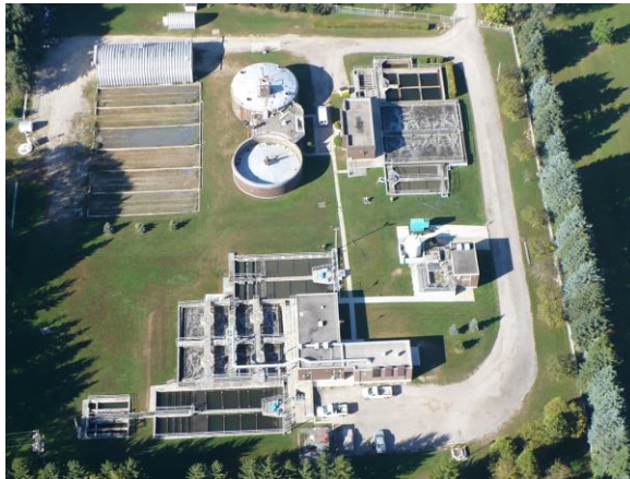
Figure 1 Aerial view of Ingersoll WWTP
