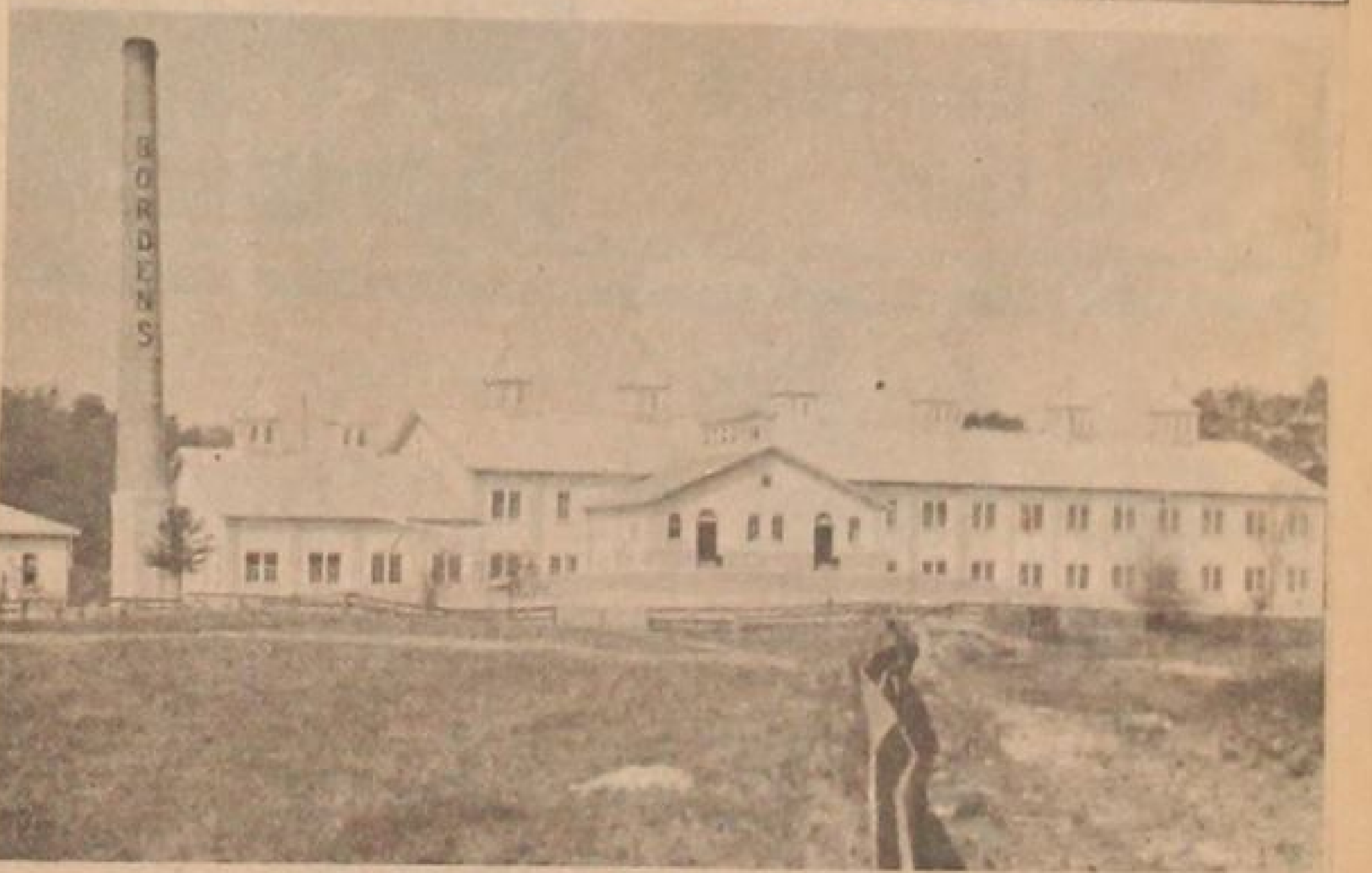
Building the condenser factory.
