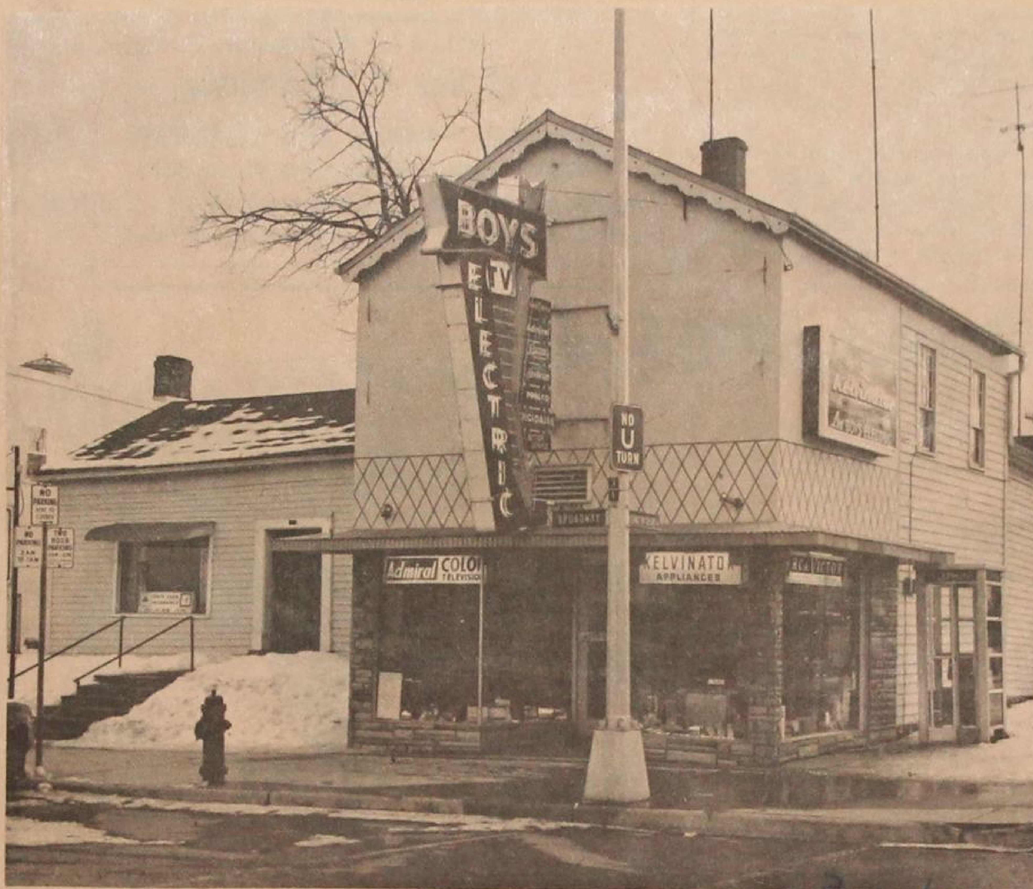
This landmark will disappear next month to make way for a modern bank building to be occupied by The Bank of Nova Scotia. Included in the plans will be a new store for Boys Electirc, who have occupied the corner for 23 years. The Boys firm will temporarily move to the Charters building, located at the north end of Broadway. Mar 172
