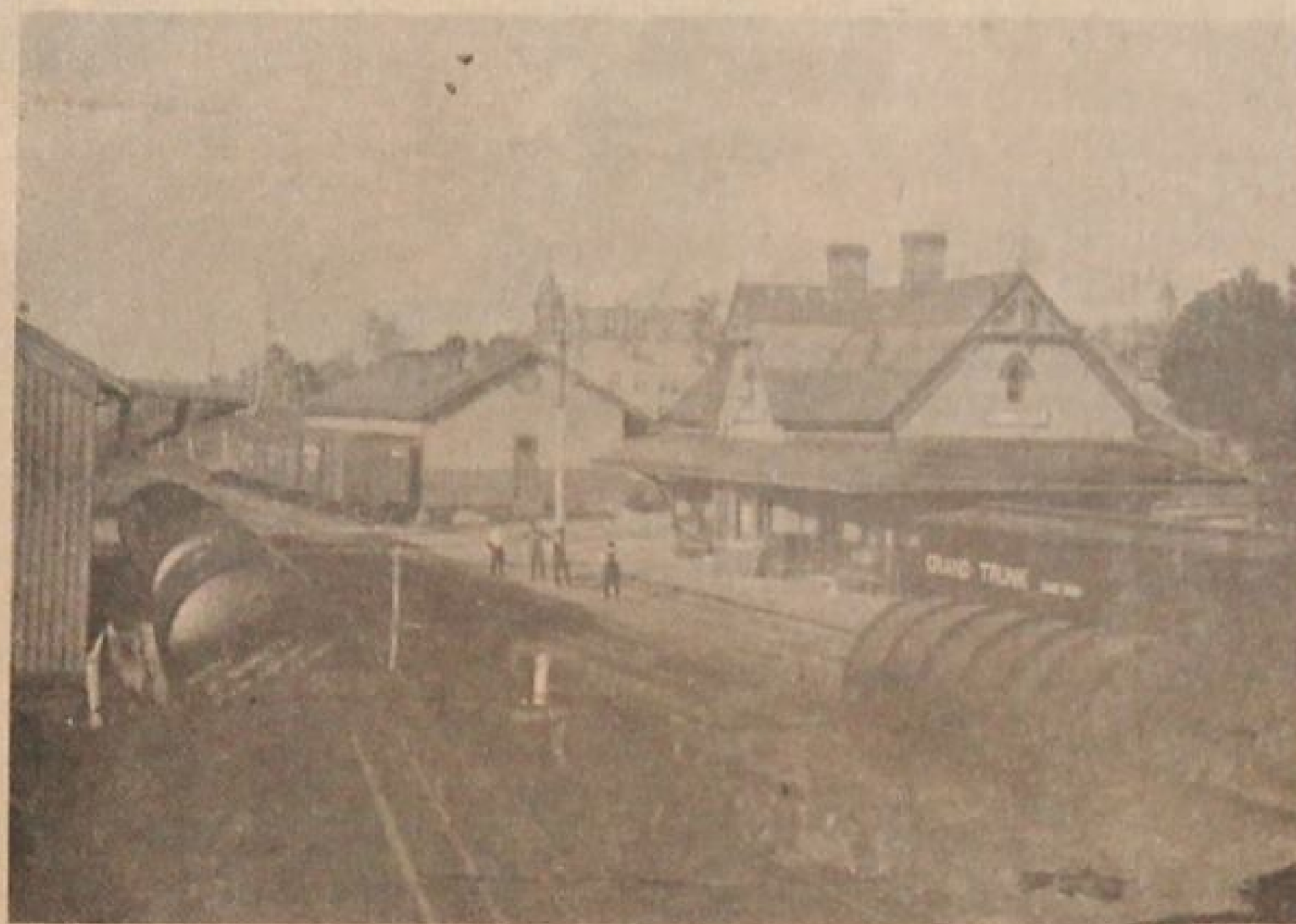
Station and sheds along Hale St.
