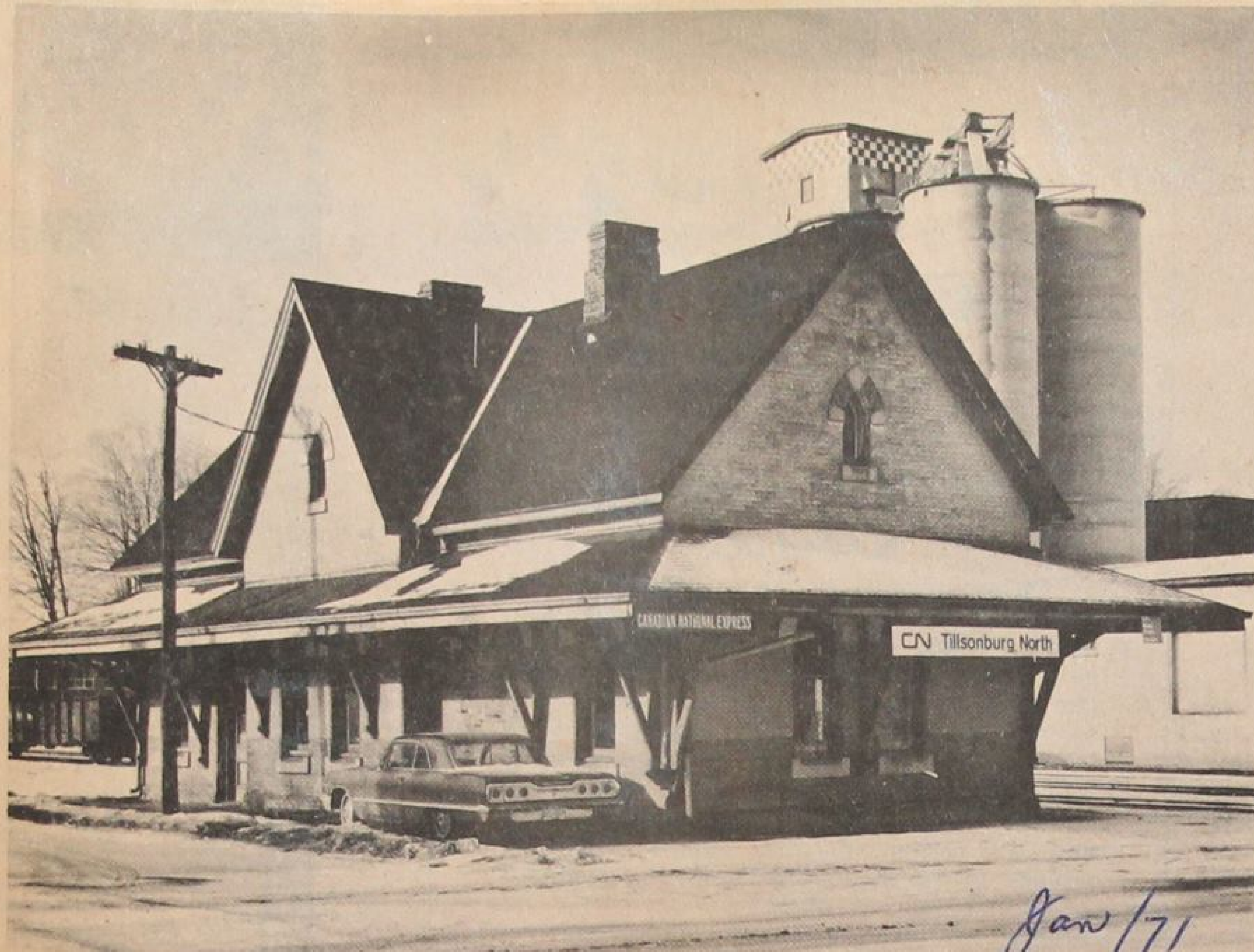
Another old landmark, the CN station at Hale and Bidwell, may soon disappear. Canadian National advised council recently that they have made application to close the station and move operations to the Wabash station on Vienna Road.
