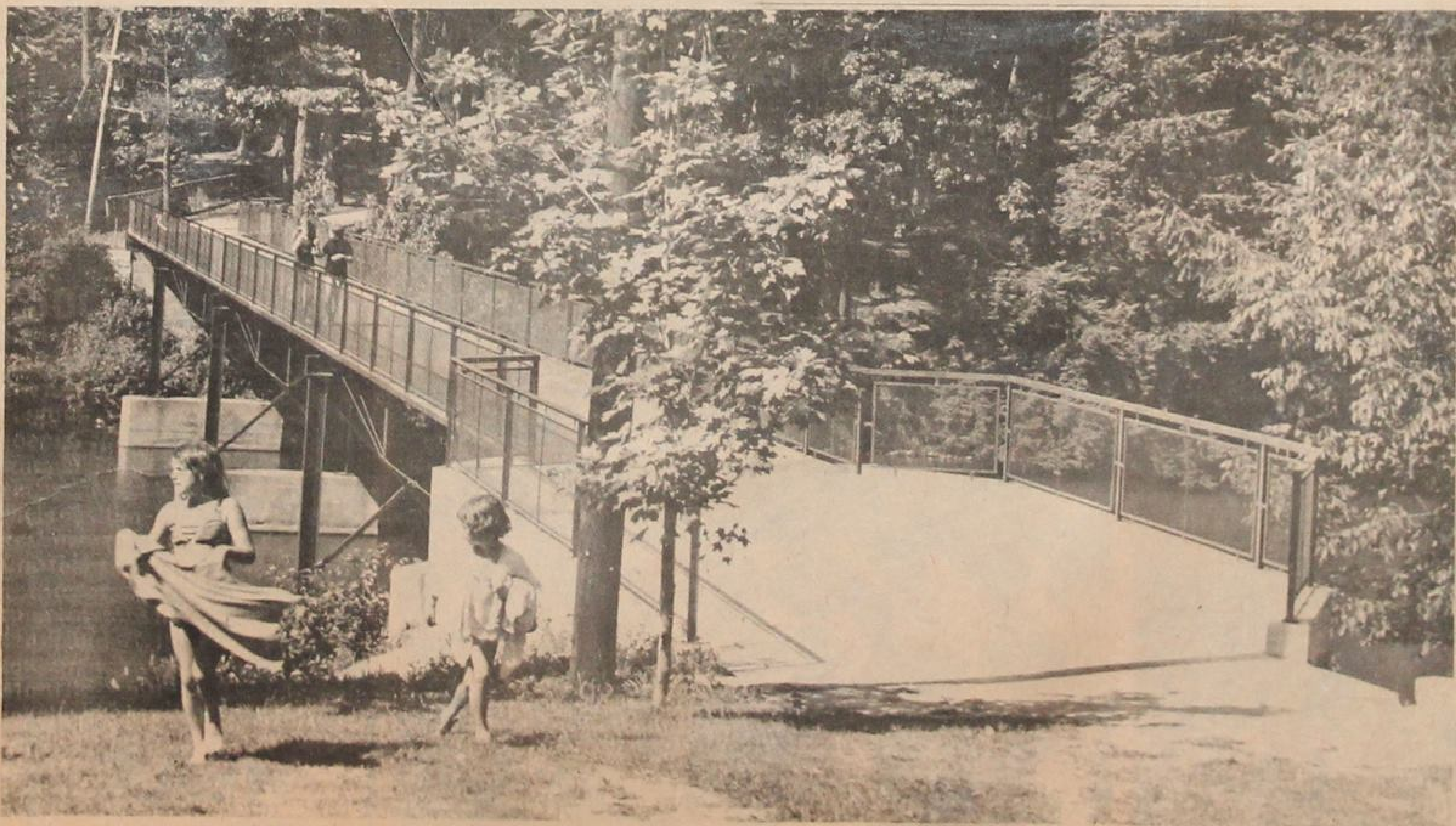
This 200 foot long, ten foot wide steel bridge is the only public access to the Otterville Lions Park. The bridge was completed in May by the Otterville Machine Shop. It was built for McMULLON'S
