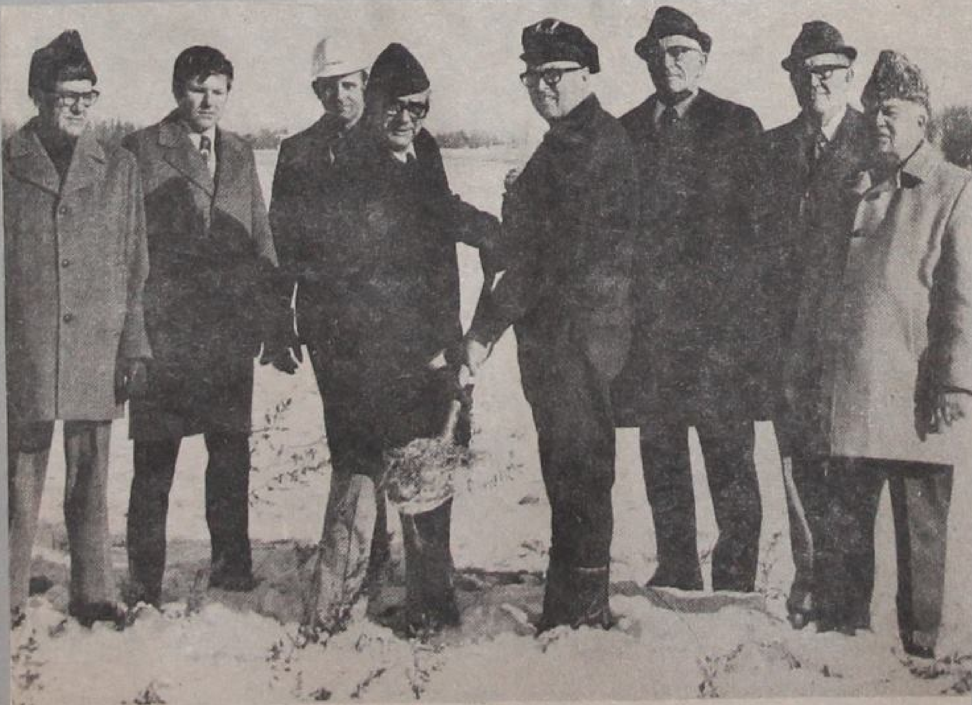
Tuesday, marked the turning of the first sod for the Norwich and District Medical Centre. North Norwich Reeve, Darwen Scott and Norwich Reeve, Stu Miles hold the sod turning shovel while other officials watch. From left are Lorne Parker, chairman of the building committee; Lenord Dickson, architect designing the new building; Harry Van Gorp, contractor; Mr. Scott, Mr. Miles, Cecil Mingle, deputy-reeve of North Norwich, Dr. Russ Hall, building and administration committees, and Eric Mannell, secretary of the two committees. Feb/1974
