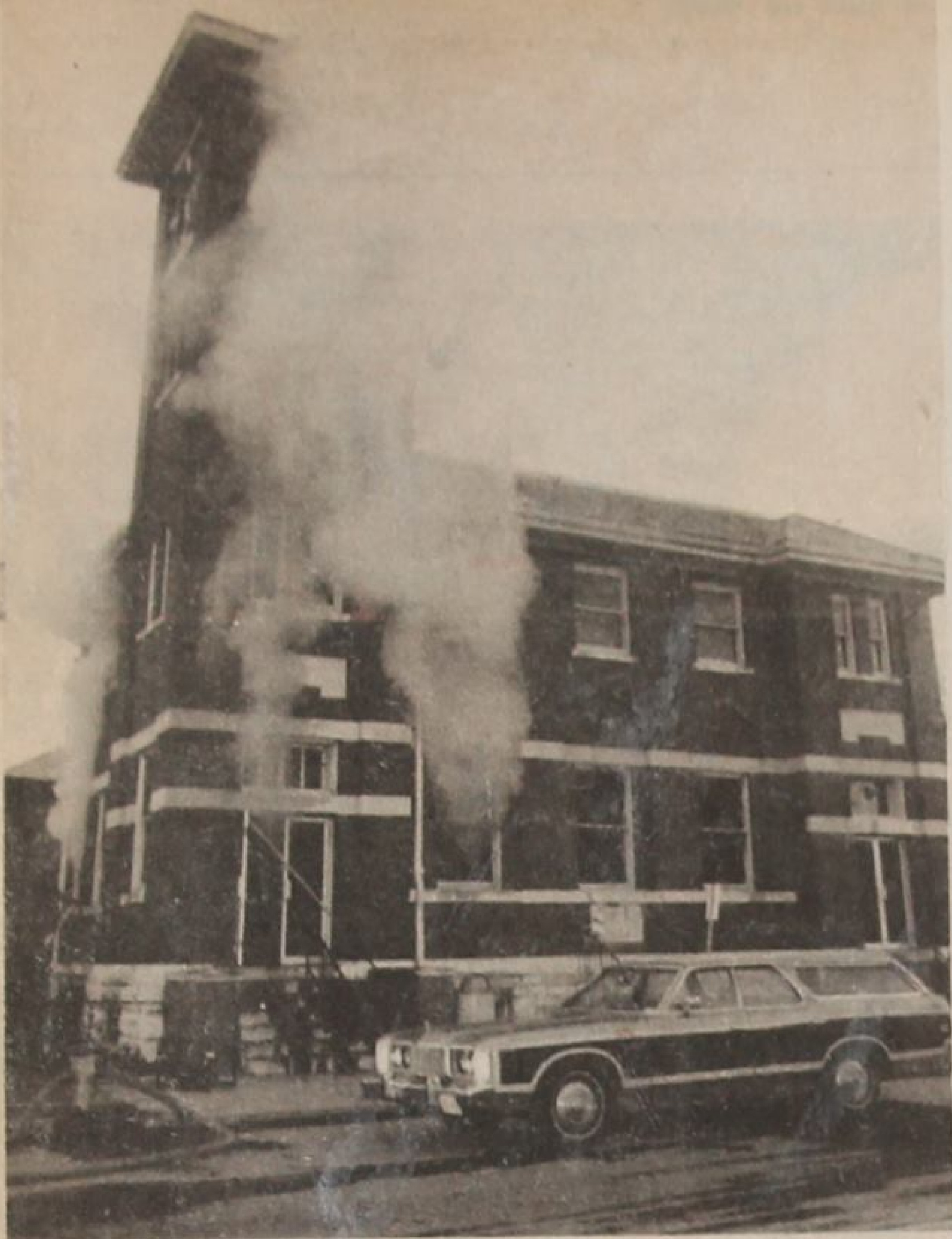
Most of the main floor area of Norwich's Post Office was destroyed by fire last week and other rooms suffered extensive smoke damage. Cause has yet to be determined but is believed to have started in the heavy double floor. The building was built more than 50 years ago and at one time housed a Canadian Customs office. (News-Record Photo)
