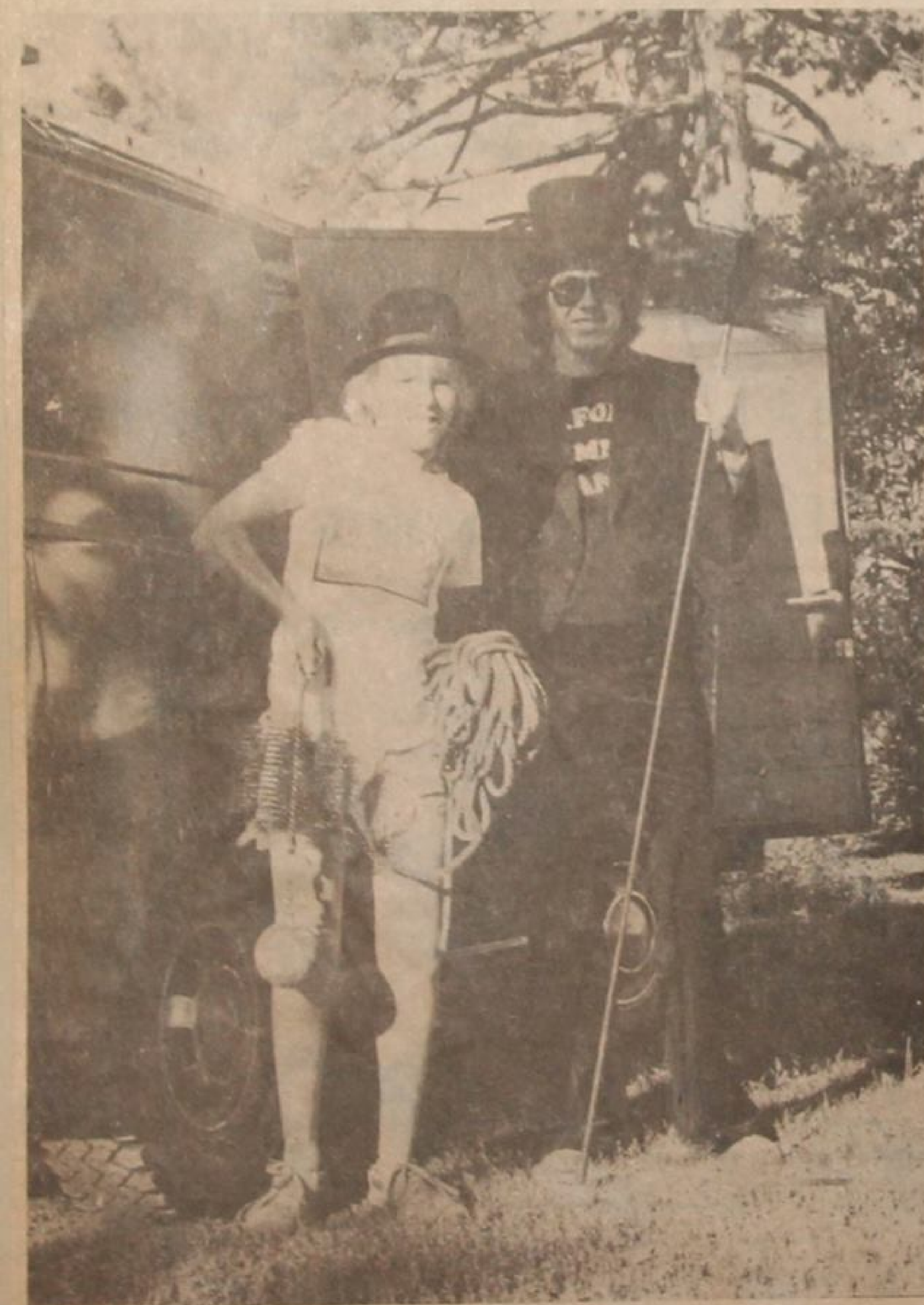
Assistant chimney sweep Paul Van den Borre and chief sweep Steve Van den Borre stand beside Steve's van. Dressed for a day's work, Steve holds a wire bristle brush coupled to the end of a fibreglas rod. Brother Paul holds a less modern tool of the trade, a weight attached to a brush attached to a rope.
