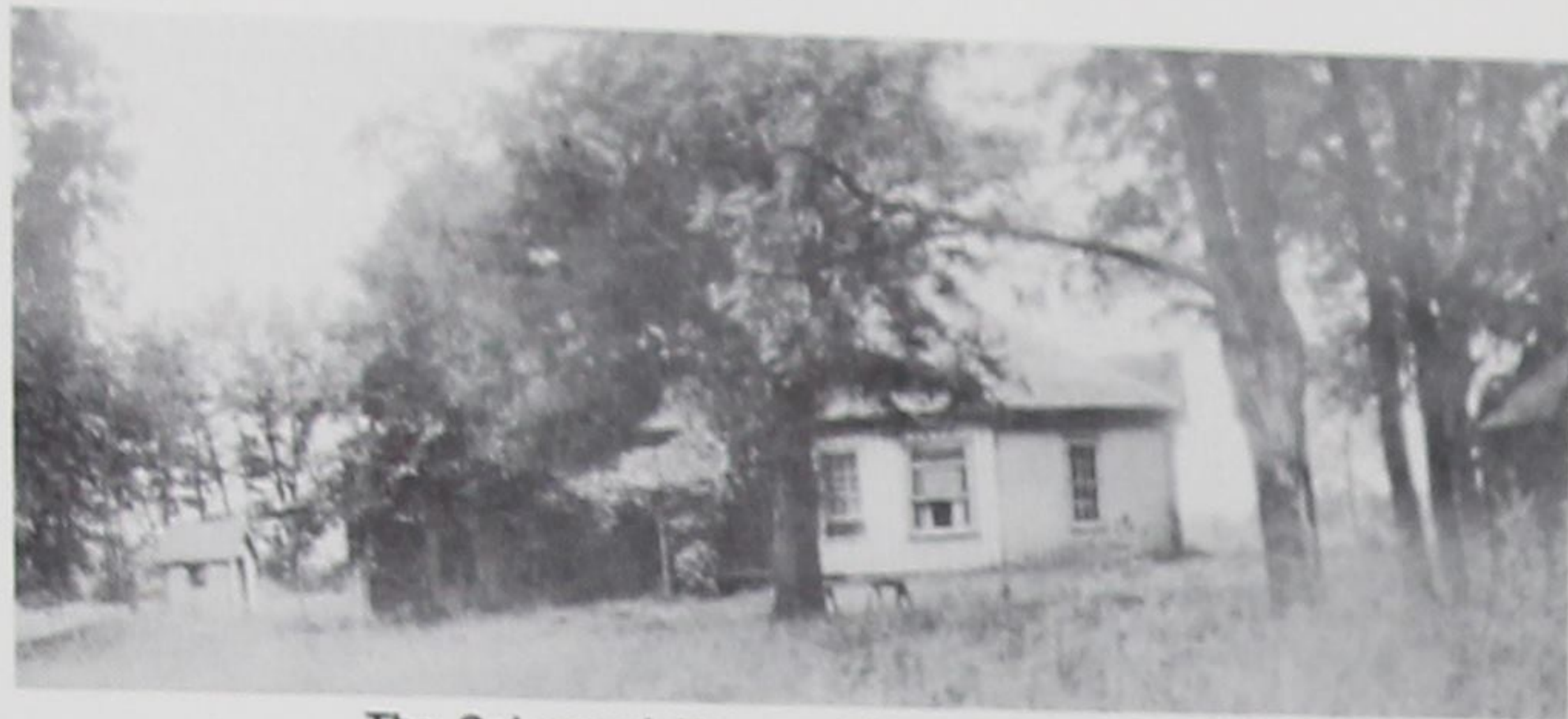
The Octagonal House at its original site.
