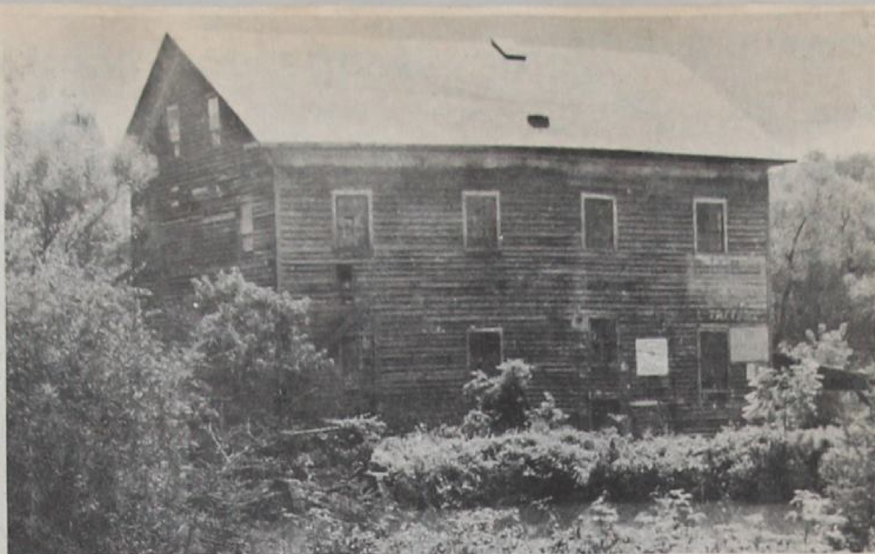
The mill is located along the Otter Creek, south of Main Street.
