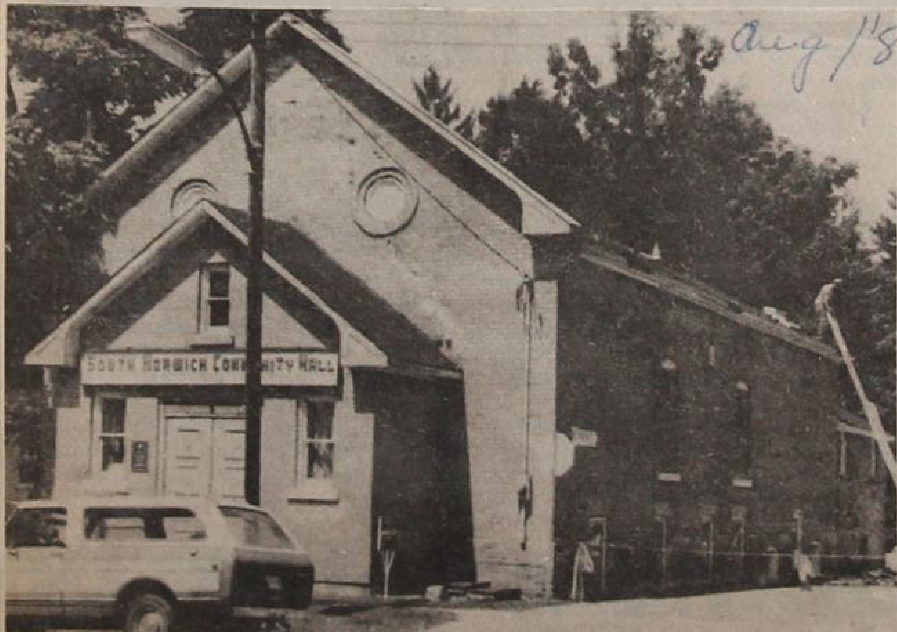
A new roof is just one of the many renovations to be completed this year at the South Norwich Community Hall, in Otterville. The hall has been used extensively since it was built by the Sons of Temperance in 1864. The village library is still located in the basement of the building which will now accommodate wedding receptions, banquets, public meetings and other local get togethers. (Staff Photo)
