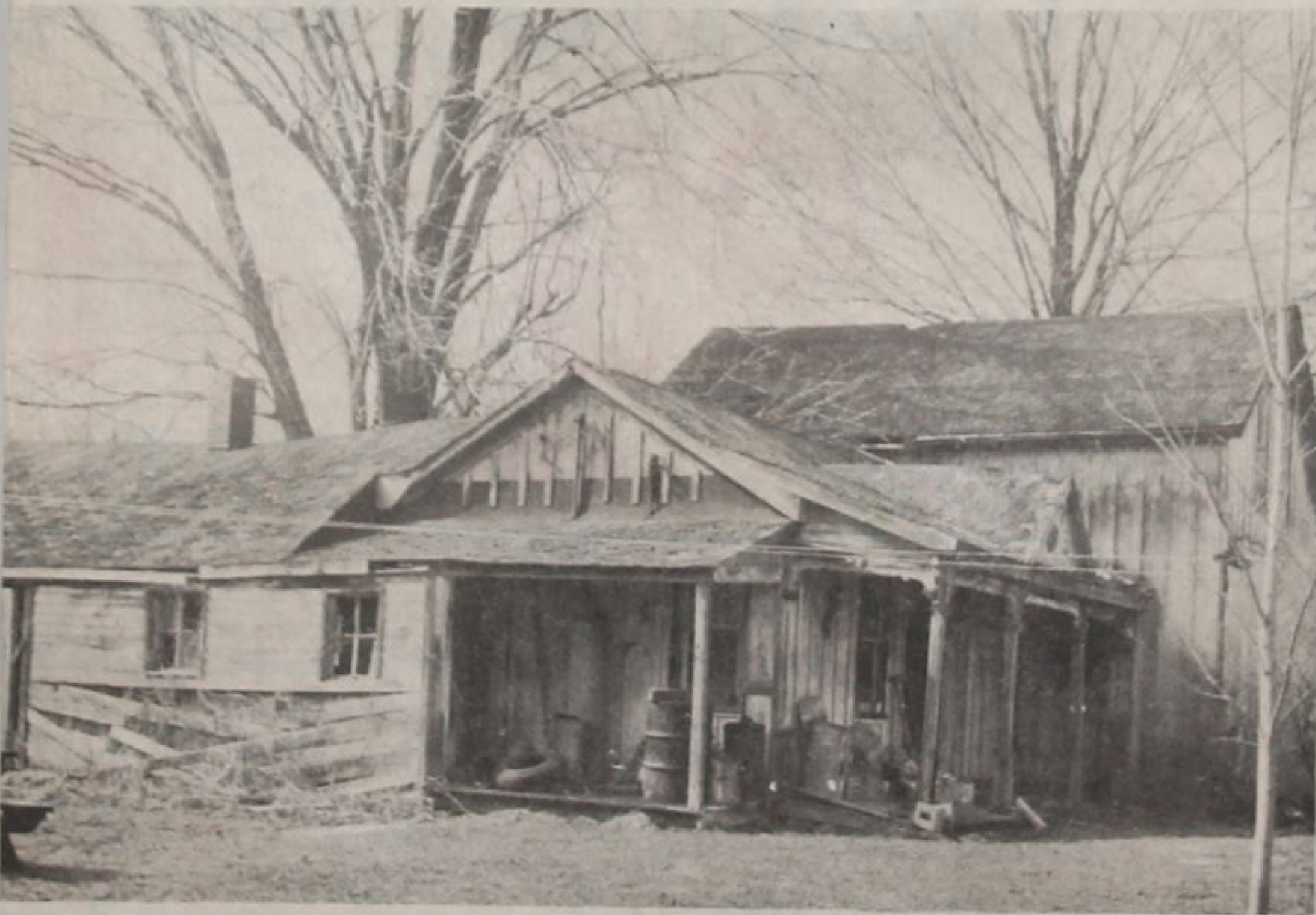
Board and batten construction and carving on the porch lintels can be seen in this weathered pioneer
