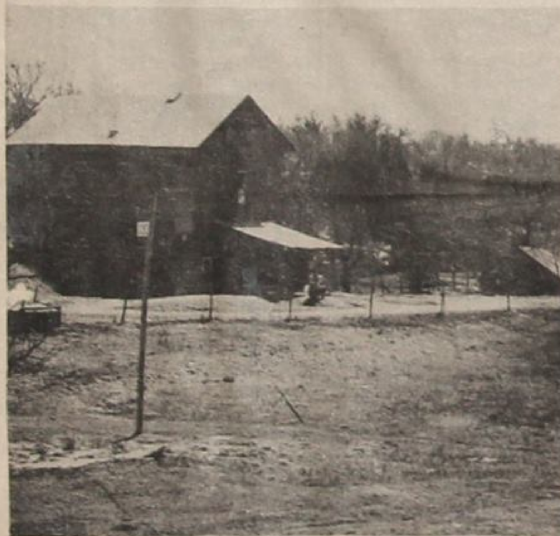
The Treffry mill, built in 1845, is one of the few authentic mills of its kind left in the area. Residents of Otterville appeared before the Township of Norwich council on Tuesday evening to enlist council's support in encouraging the Long Point Region Conservation Authority to purchase and preserve the property.
