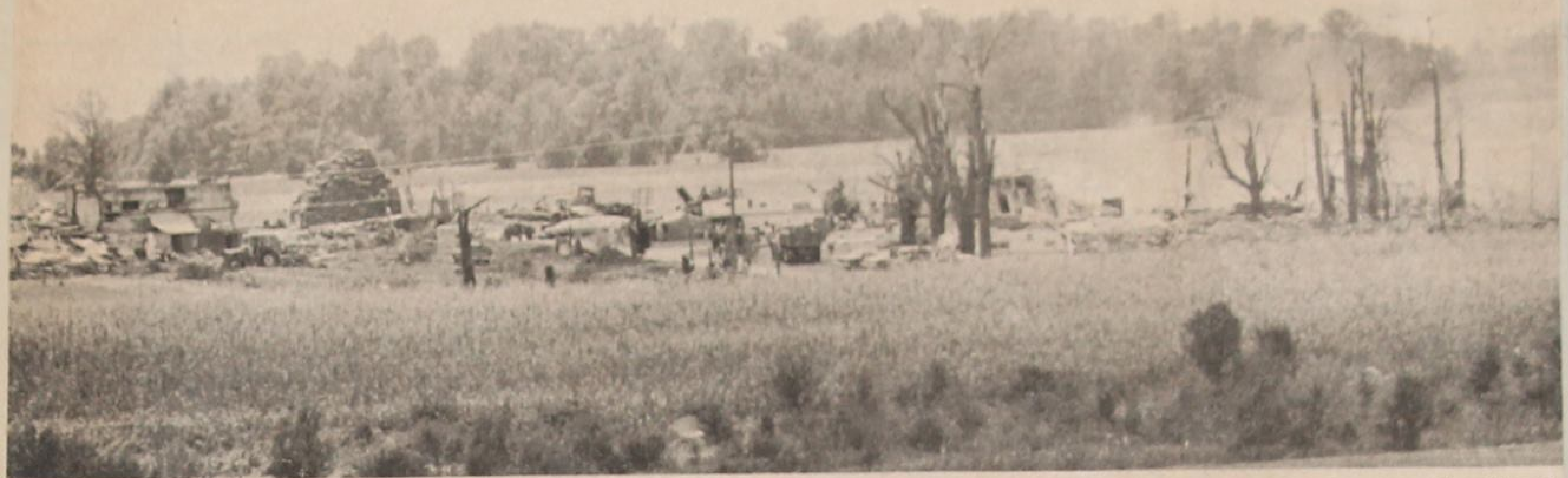
On a hill overlooking these farms just south-east of Oxford Centre, the path of destruction of last Tuesday's tornado can be seen. Buildings in the direct path of the tornado were literally razed, trees broken off or uprooted entirely and vehicles swept up to be found
