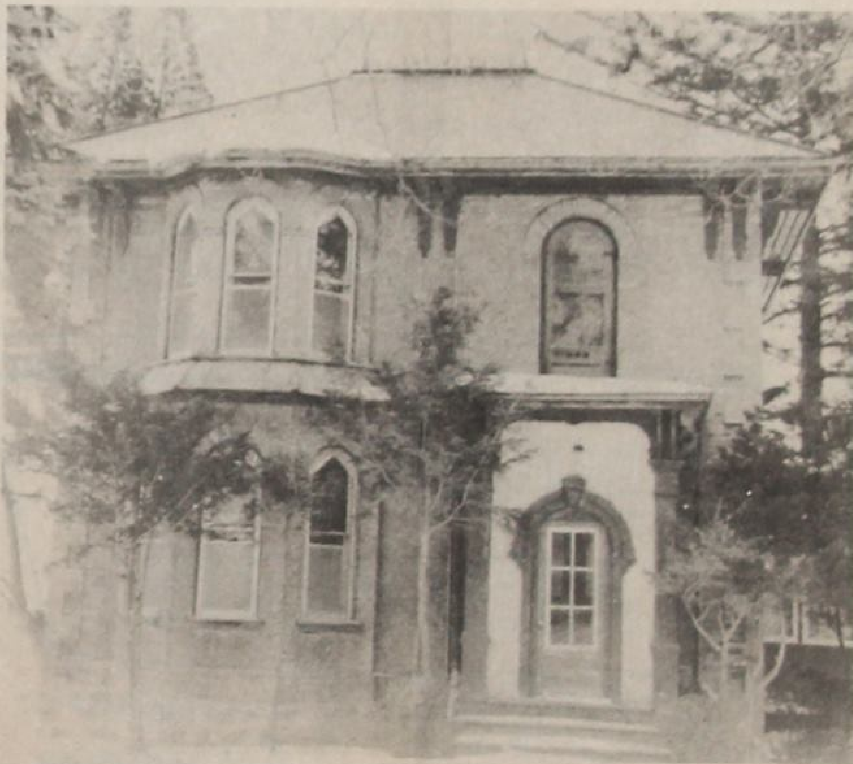
According to "With Mortar and Pine", a book compiled by the Local Architectural Conservation Advisory Committee, the Italinete style was very popular in the 1860's and 70's. A massive square shaped and high pitched roof are indications of this style. (News-Record Photo)
