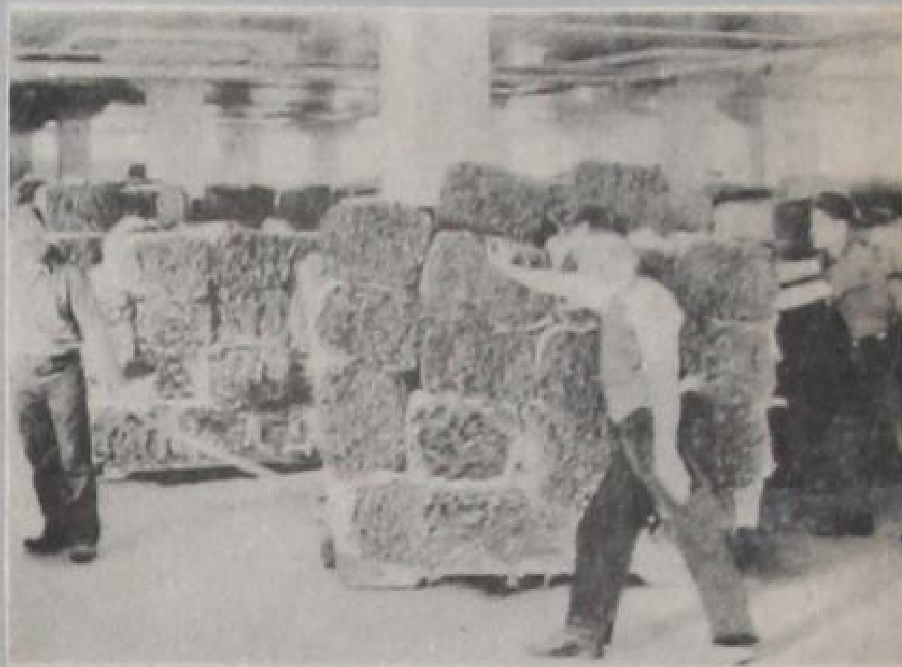
Storing of baled Tobacco, awaiting grading.
