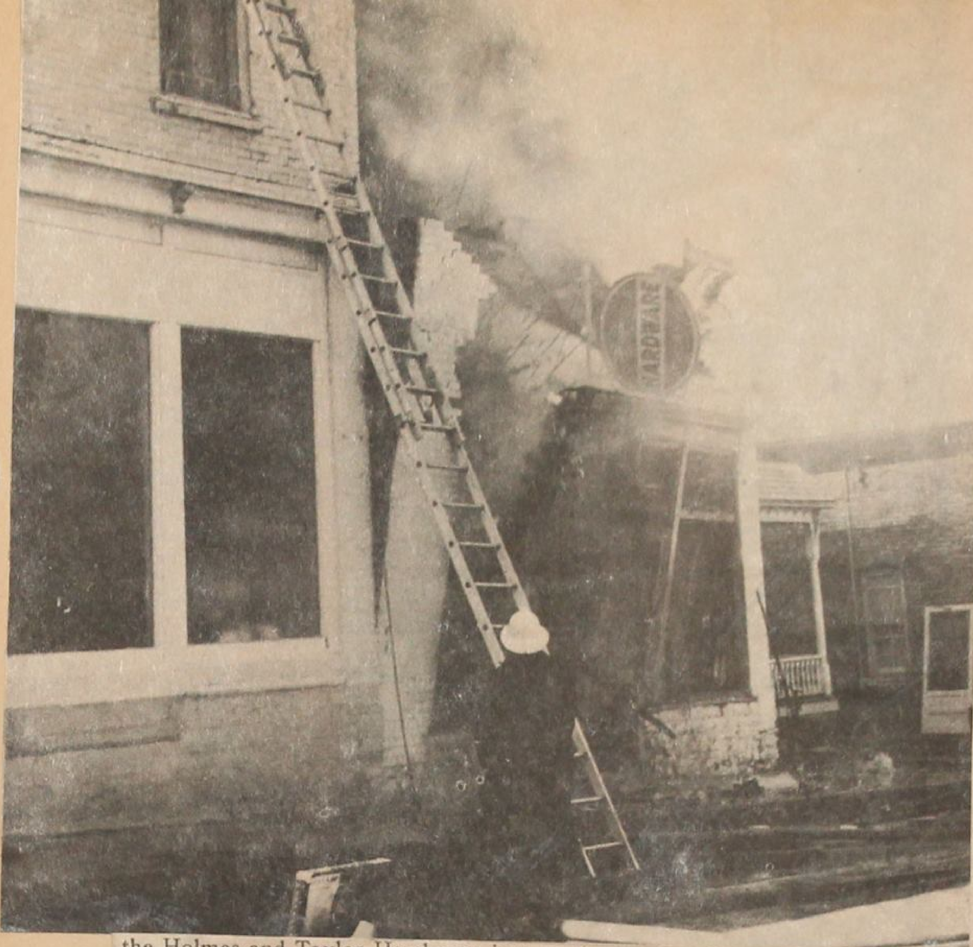
the Holmes and Taylor Hardware just as the front wall started to fall
