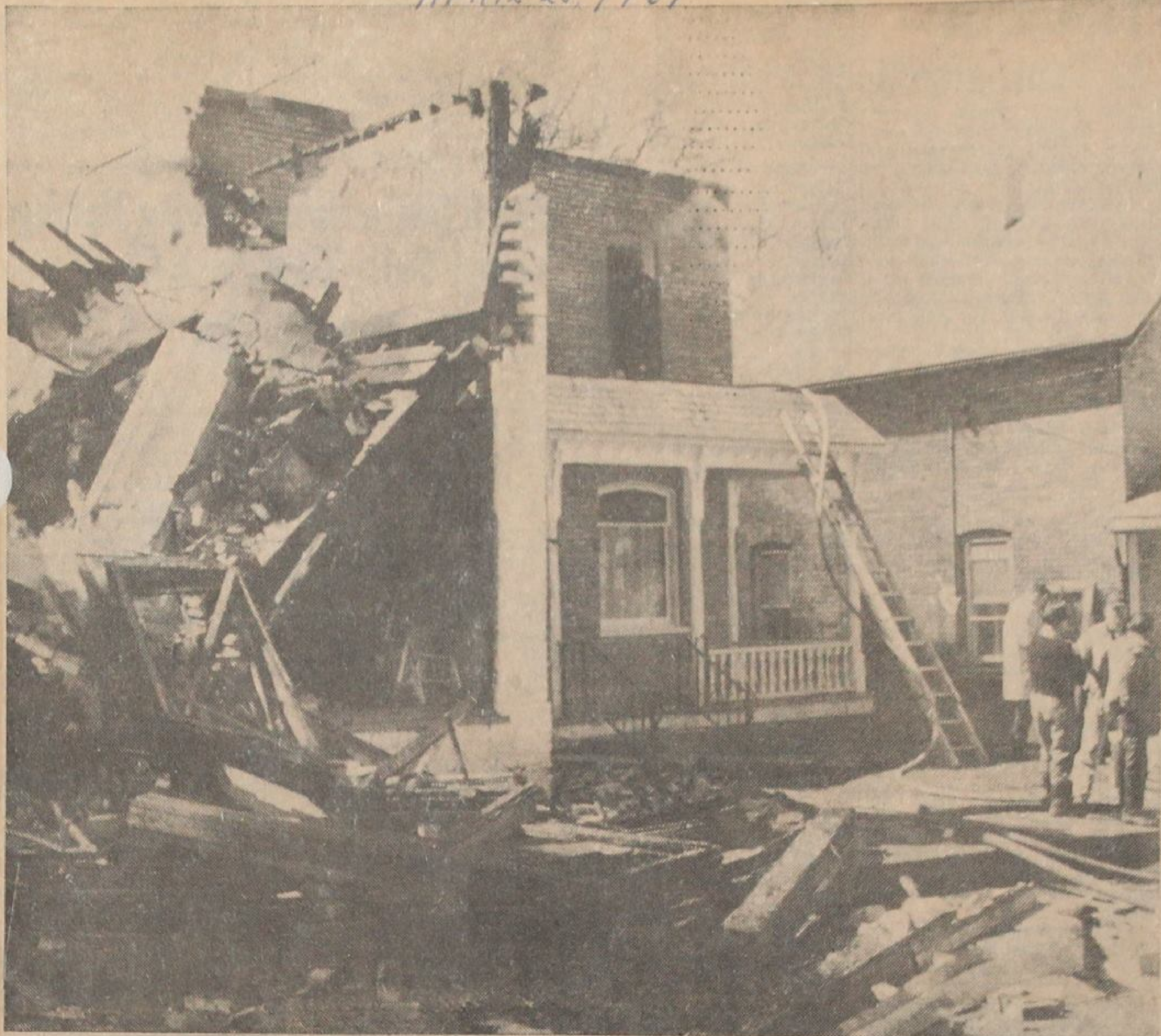
THE RUINS of the Holmes and Taylor hardware and appliance store, destroyed by fire in Otterville this morning, are seen at the left of this photo. The home of one of the owners, Murray Holmes is on the right. The residence, with the walls still standing, was completely gutted. Firemen and neighbors managed to save a few items of furniture from the home.
