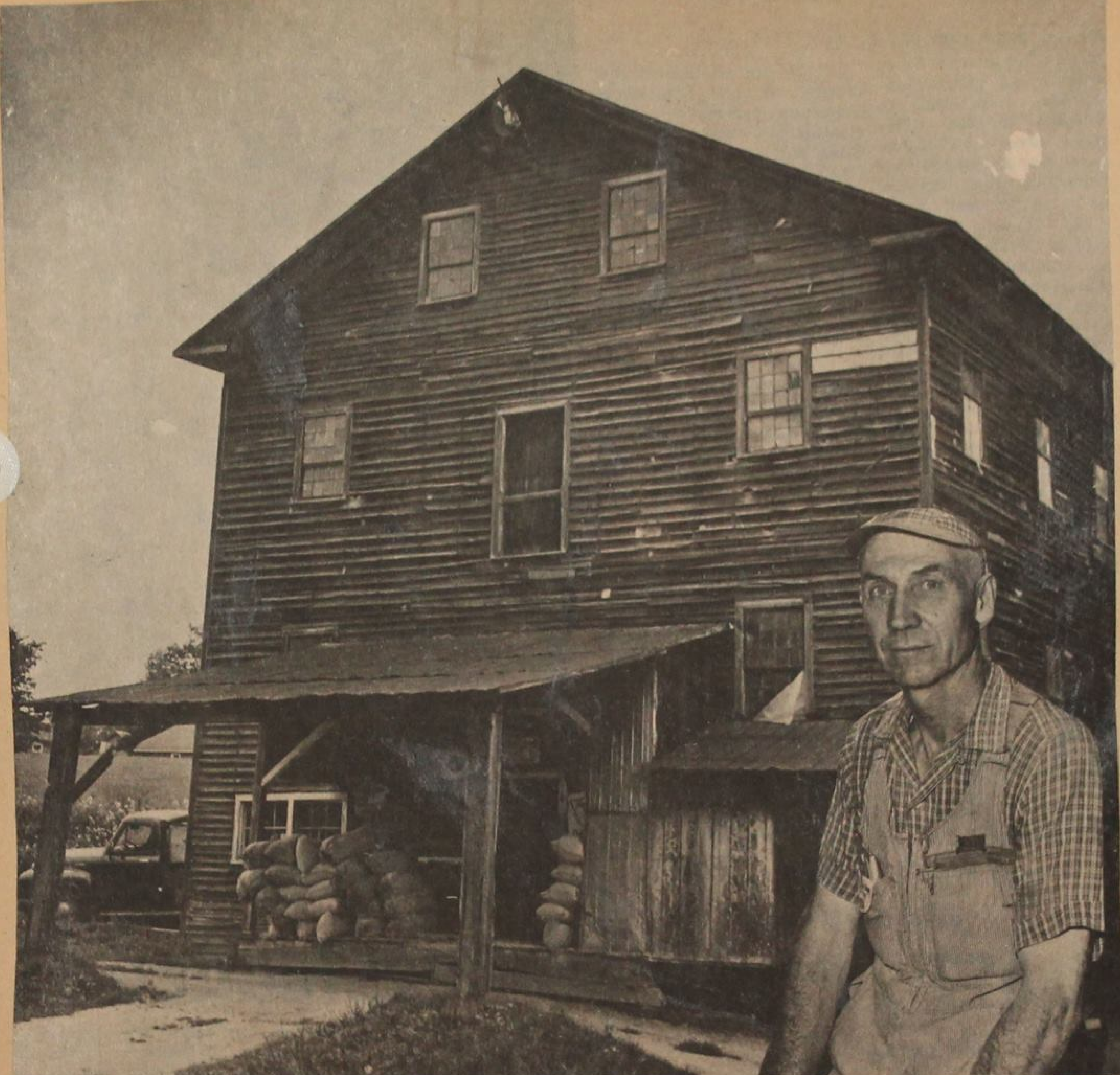
A historic old building in the Village of Otterville is the grist mill, located just off Main Street. It is still in operation, after being a "going concern" for the past 122 years, its source of power, the pressure of water against a steel turbine, that makes it one of the few grist mills around using water power. It is owned and operated by Lorne Treffry of Otterville, shown at bottom right, who purchased it from his father, Ernest Treffry, in 1952. (Photo by Ellen H. Eff)
