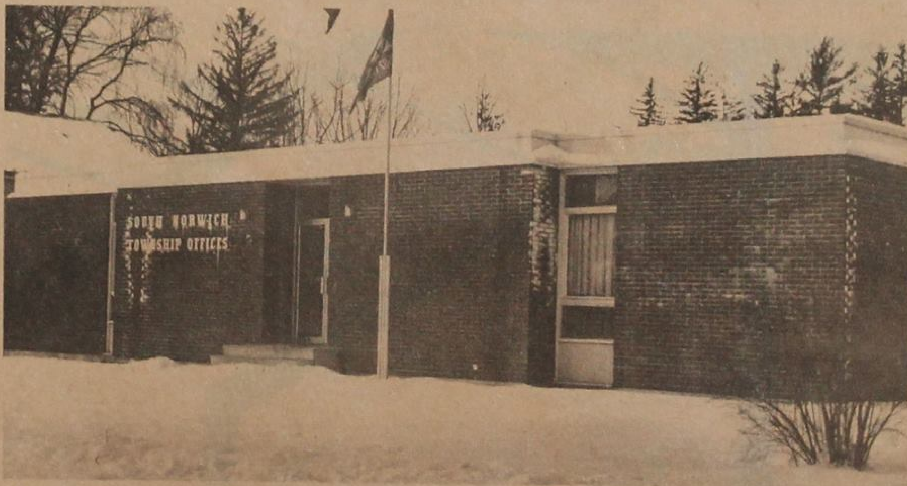
The handsome new township office building, located in Otterville, was a centennial project for South Norwich Township. A museum is housed in the basement of the building.
