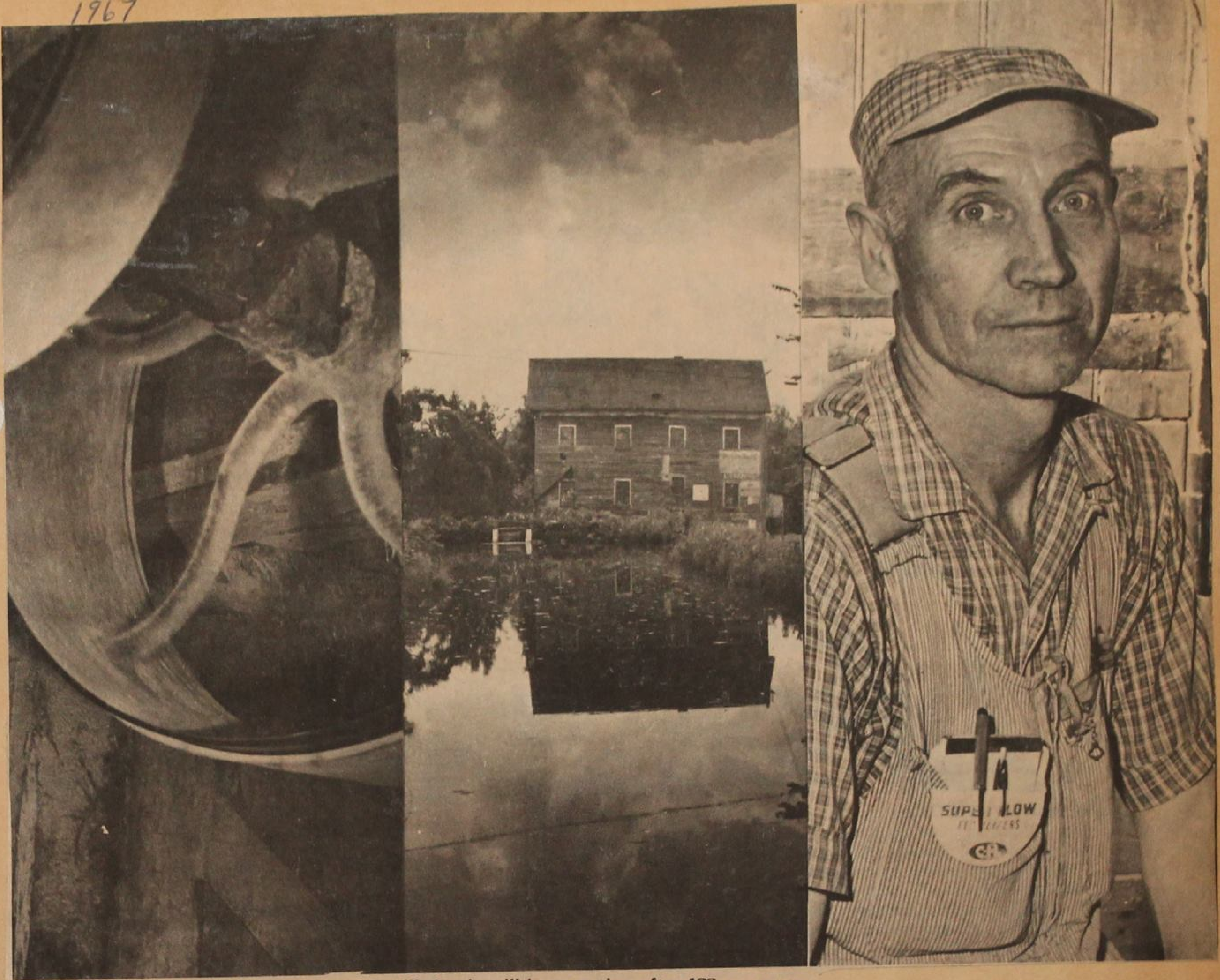
In the Village of Otterville is an old grist mill that is still in operation after 122 years, its source of power that grinds the mixed feeds the pressure of water against a steel turbine, shown at left. Secondly on view is the mill, located south of the main street, on a site where there has been a mill since 1870. Third from left is pictured the owner and operator, Lorne Treffry, who took over the operation of the grist mill from his father, Ernest Treffry, in 1952.
